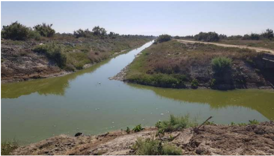
Figure 15: Views of the second range drainage channels in the project area
