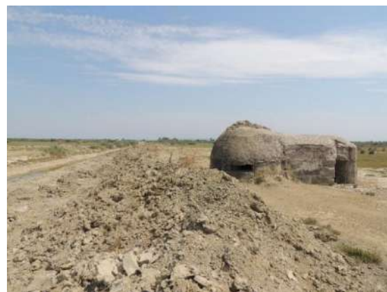
Figure 29: Bunker along drainage channel
